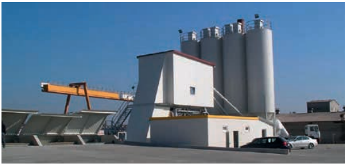
Row-type silo plant with below ground concrete silo
