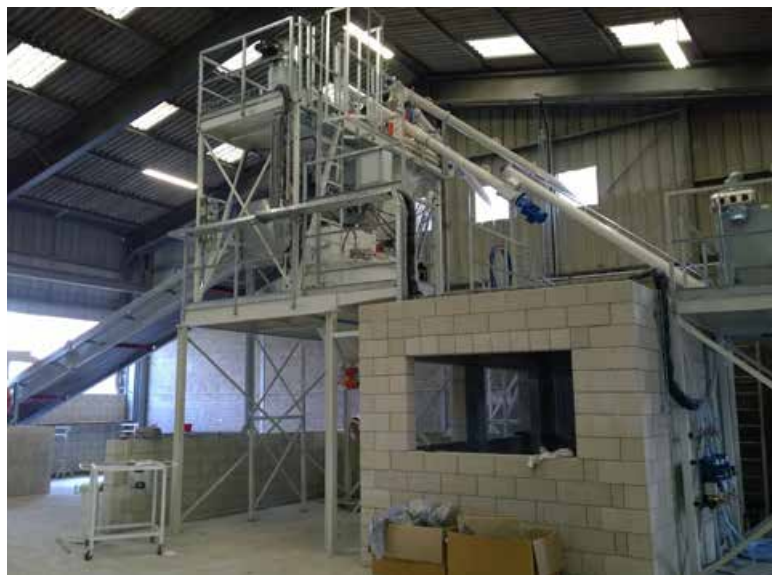
Special mixing plant for UHPC
