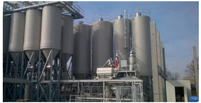
Row-type silo plant with 34 aggregate silos for architectural concrete
