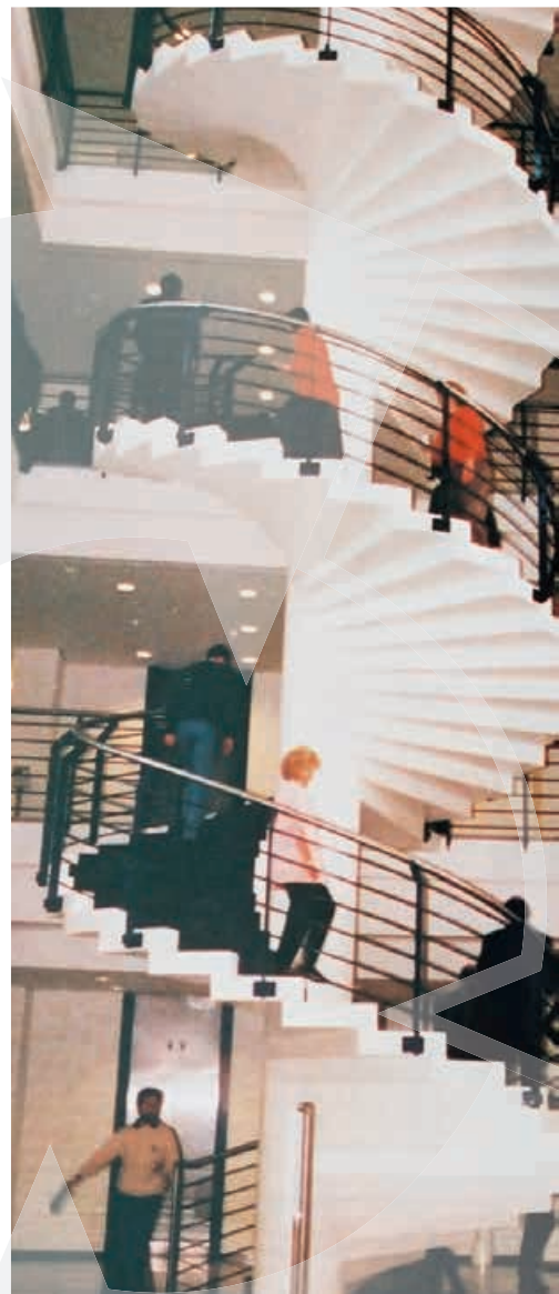
Concrete spiral stairs
