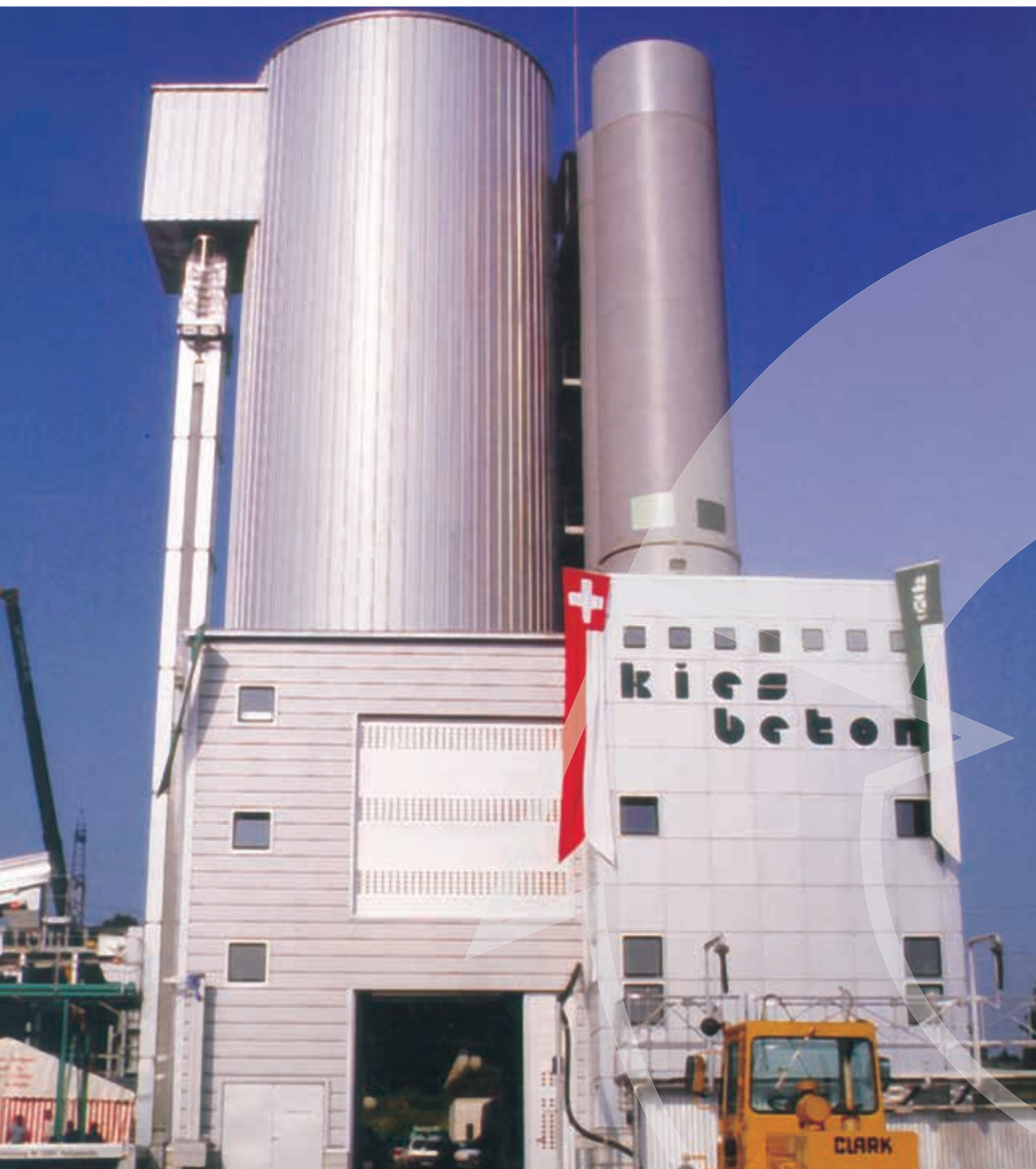
Tower plant with a capacity of 520 m 3
